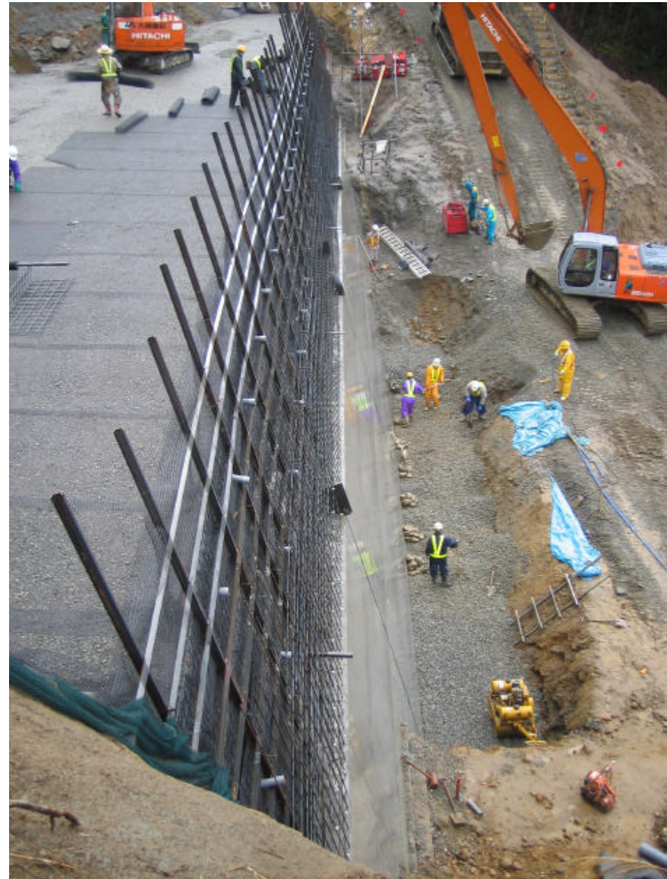
2) PLACING GEOTEXTILE AND GRAVEL GABION
