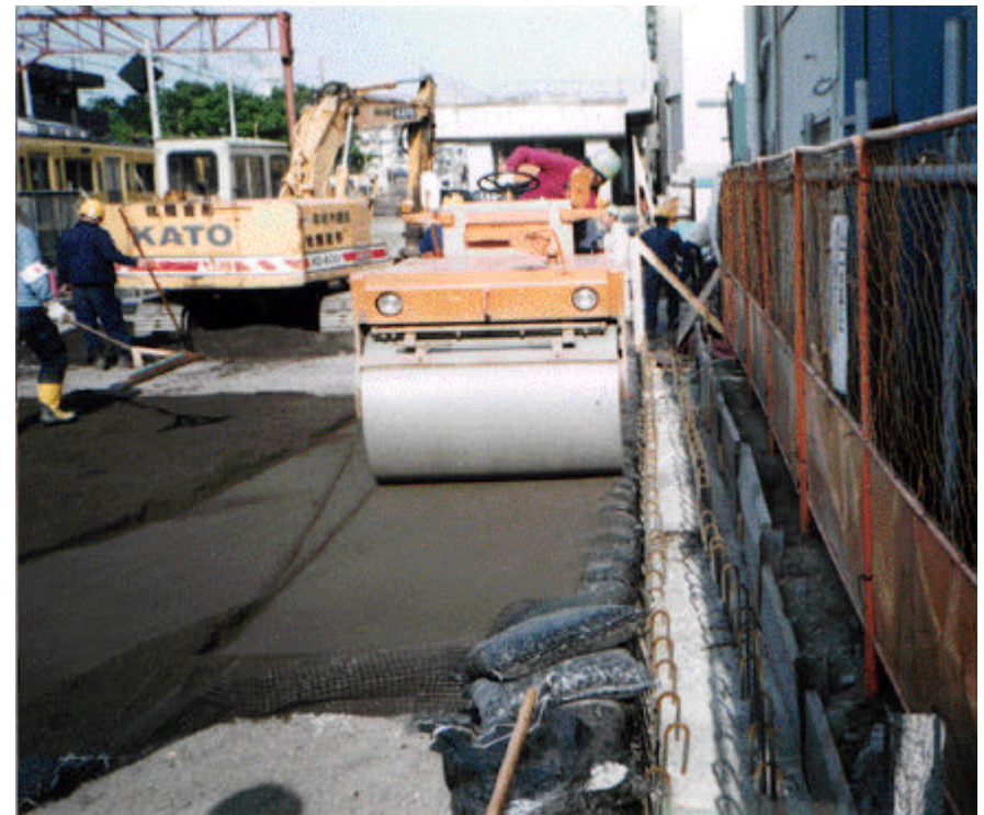
2) PLACING GEOTEXTILE AND GRAVEL GABION
