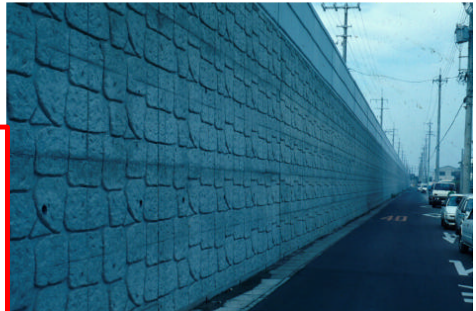
6) CASTING-IN-PLACE OF RC FACING
