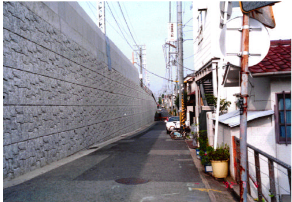
Reinforced-soil RW having a full-height facing at Tanata site
