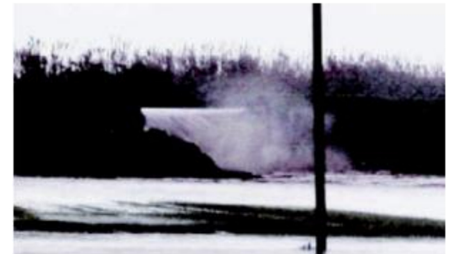
District of Pisa: piping phenomenon through the embankment (landside over the river bank). From "La voce del Serchio".
